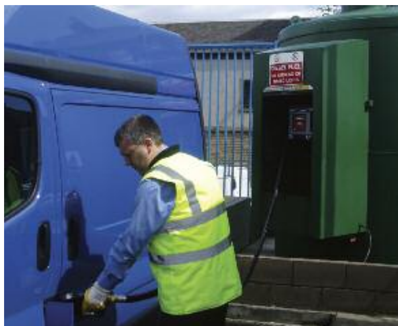
The Titan FuelMaster 10,000 litre capacity tank
