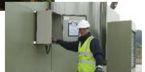
Checking levels in Countrywide's new storage facility at Weston super Mare
